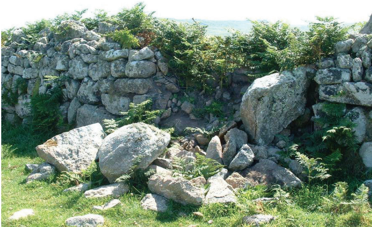
Fig. 3.6 Collapsed Penwith hedge. The quick and cheaper option of fencing often results in stock proofing of outer field boundaries, reducing the need to maintain internal field boundaries. © Cornwall Council HER
